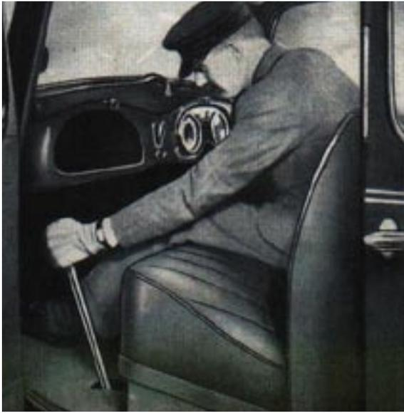
*The Ranelagh had in-built hydraulic jacking operated from the driving compartment.*
